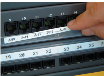
Punch block & patch panel labels
