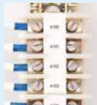
Terminal block marking
