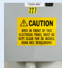
Hazard warning signs
