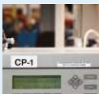
Control panel and electrical panel labels
