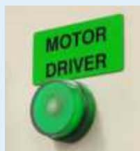
Raised panel labels
